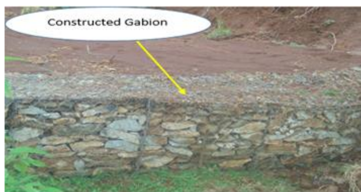
Figure 6: Gabion constructed for protection of erosion in the Gilgel Gibe watershed (Picture taken by the principal)
