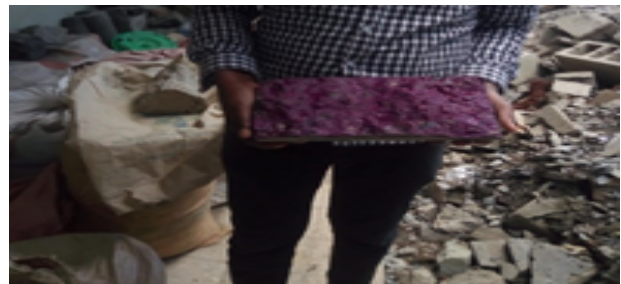
Figure 9: Concrete Exposed to Phenolphthalein Solution
